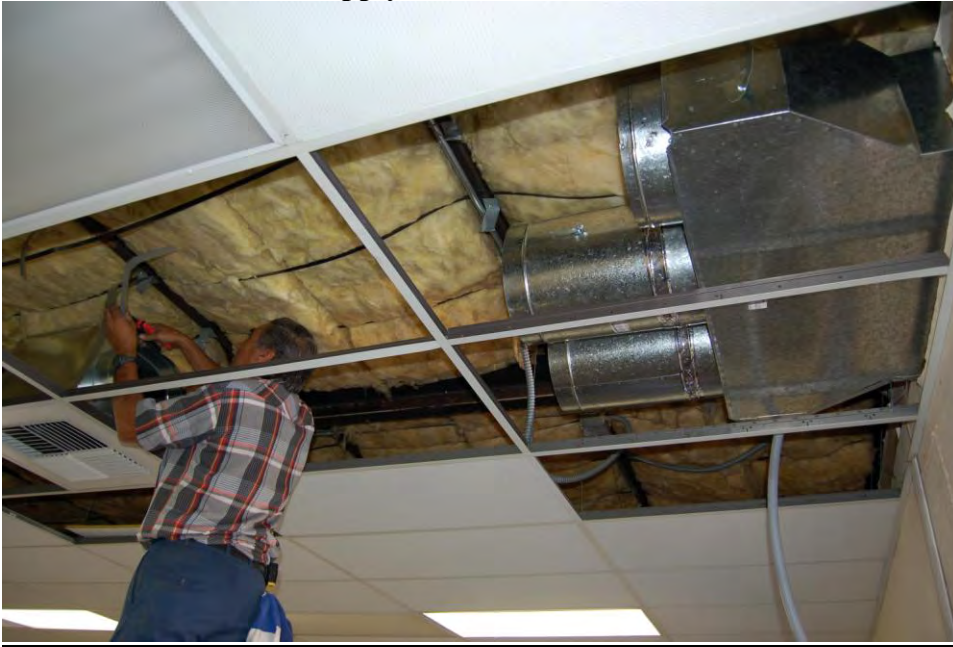
Installation of 3 outlet supply ducts
