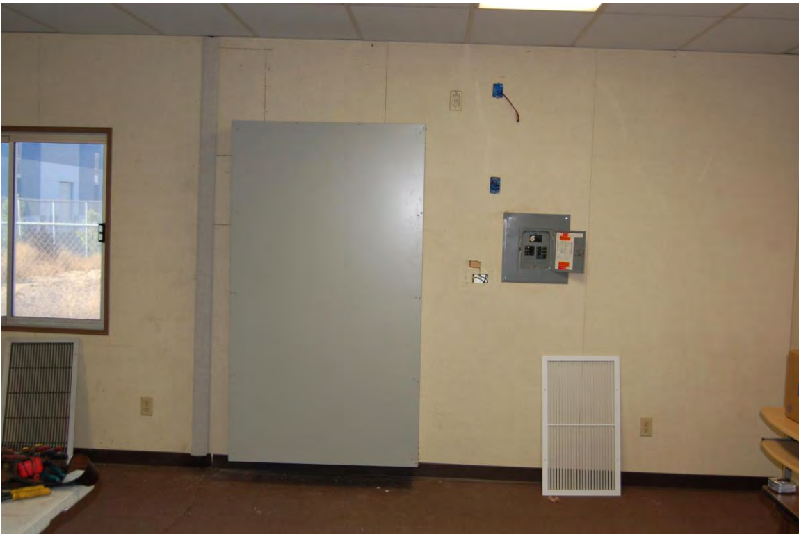
Interior with Return Air Acoustical Plenum installed.
