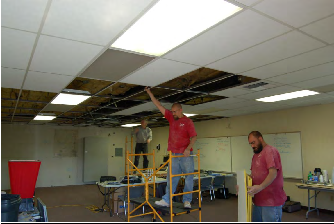
Interior with the ceiling tile being replaced.
