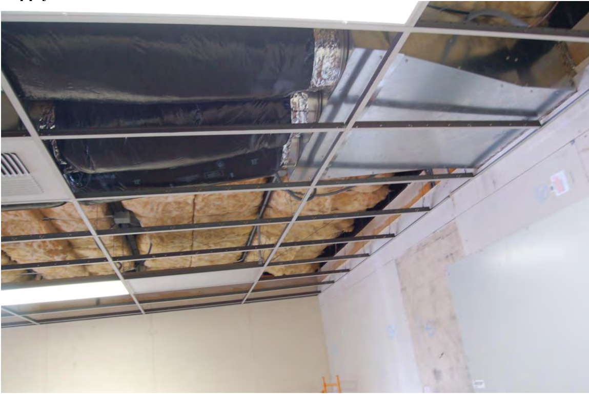
Supply Air Acoustical Plenum installed – 3 outlets.
